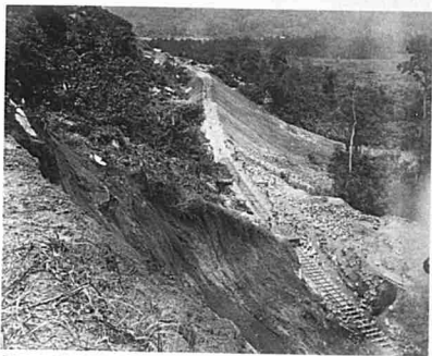
82. Work on Perak Railway at Gunong Pondok.
