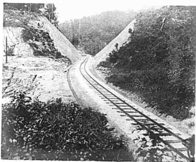
83. Newly constructed Perak Railway.
